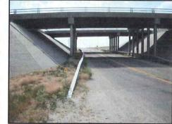
structure. In lieu of complete reconstruction of the bridges, retrofitting the road cross section with minimal shoulders should adequately serve the public as an interim measure until such time that pedestrian and cyclist use warrants otherwise.
